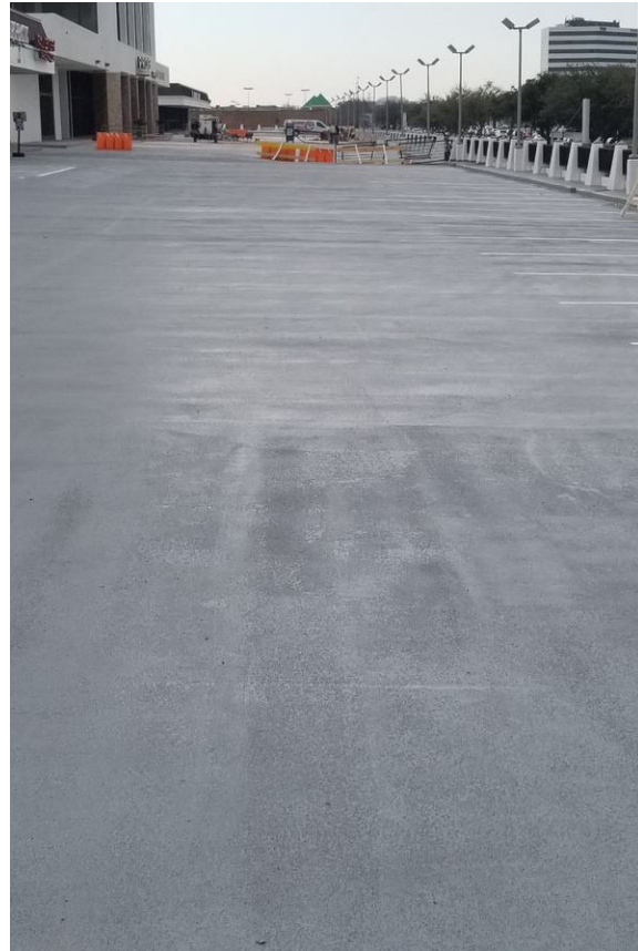
Completed concrete profile
