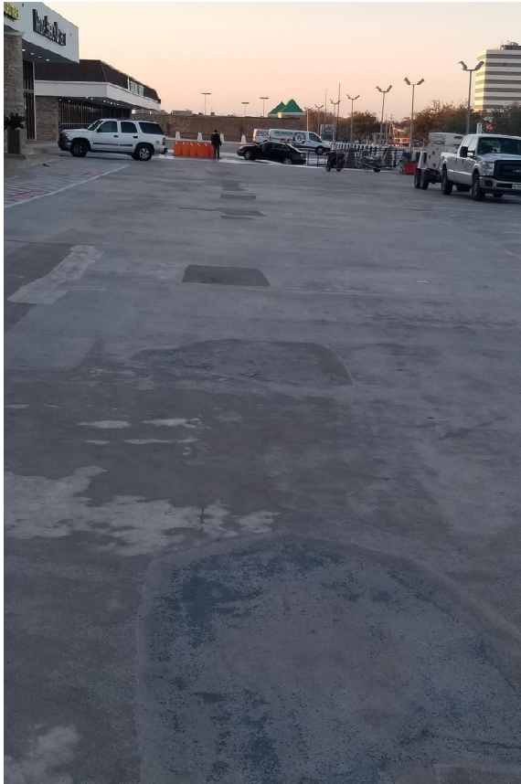
Beginning concrete profile
